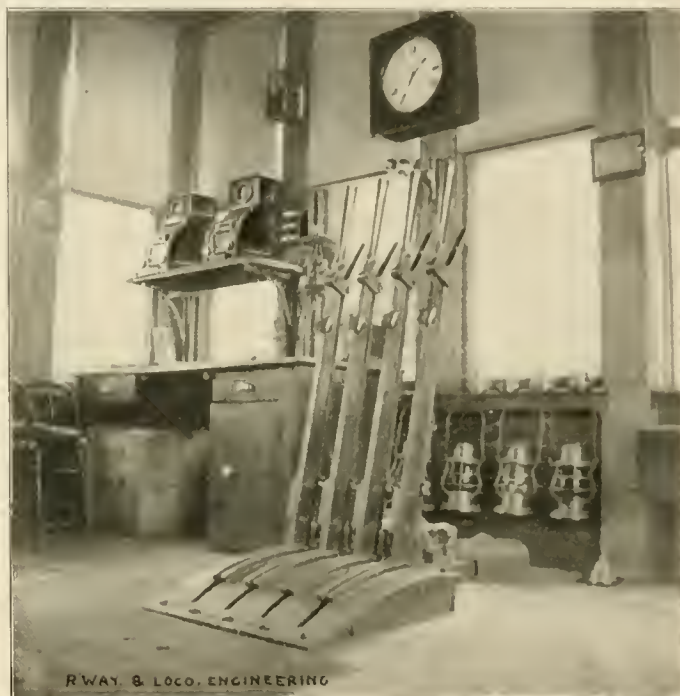
INTERIOR OF BLOCK SIGNAL TOWER ON THE NEW YORK CENTRAL RAILROAD, SHOWING SIGNAL LEVERS AND INSTRUMENTS.
